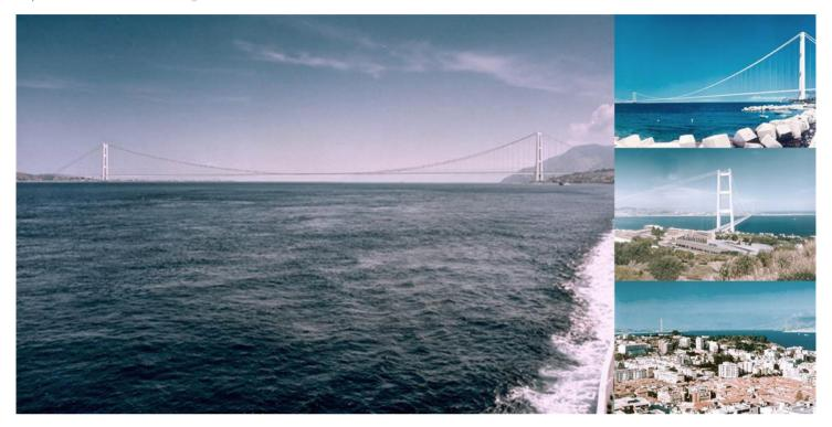
The bridge over the Messina Channel which will connect the region of Reggio Calabria, in the South of the Italian Peninsula, with the Island of Sicily, is a 3.70km long suspension bridge with a central span of 3.30km.
